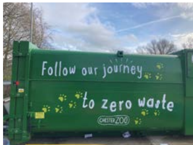
Waste compactor at Chester Zoo's new Resource Recovery Centre.
