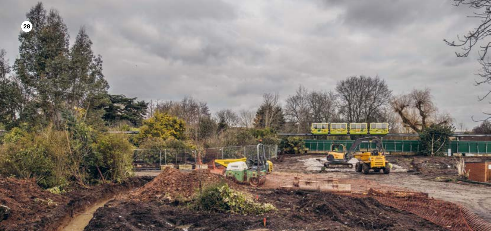
Building works for the lemur walk-through experience
